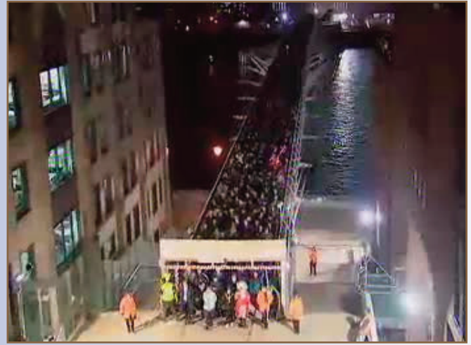
Figure 1: The London Millennium Bridge failure, due to wrong input in the FE modeling. Left: snapshot from a YouTube movie, showing the wobbling of the bridge during its opening. Right: snapshot from another YouTube movie, showing the testing of the bridge after its repair and before its reopening. Figure 3.11 in the book includes the QR codes for these two movies.
