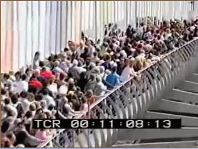
Figure 1: The London Millennium Bridge failure, due to wrong input in the FE modeling. Left: snapshot from a YouTube movie, showing the wobbling of the bridge during its opening. Right: snapshot from another YouTube movie, showing the testing of the bridge after its repair and before its reopening. Figure 3.11 in the book includes the QR codes for these two movies.
