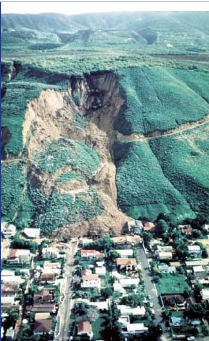
Figure 2: Rainfall induced La-Conchita slope instability, 1995 - Courtesy of USGS
