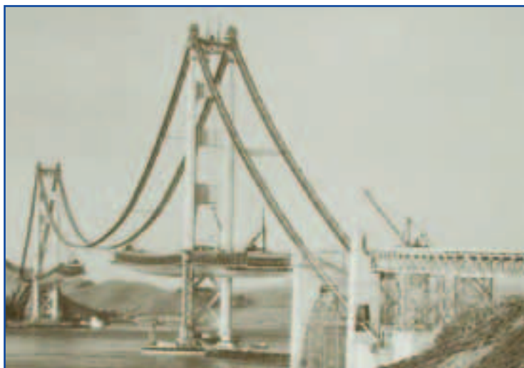
Figure 9: Manufacturing of truss girder
