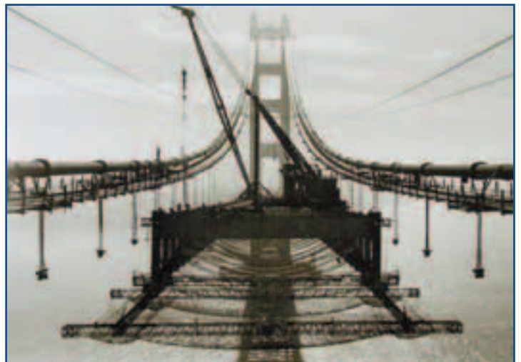
Figure 8: Erection of main girder with safety net
