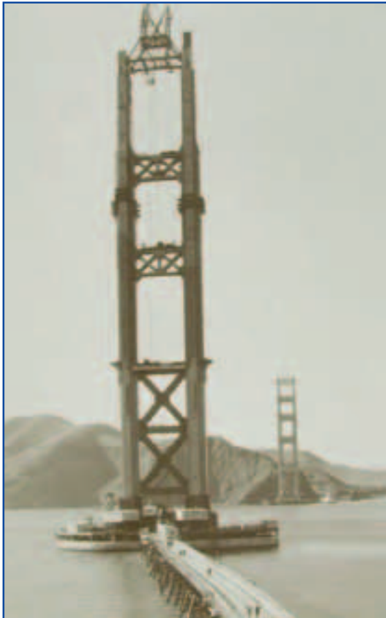
Figure 7: Erection of towers
