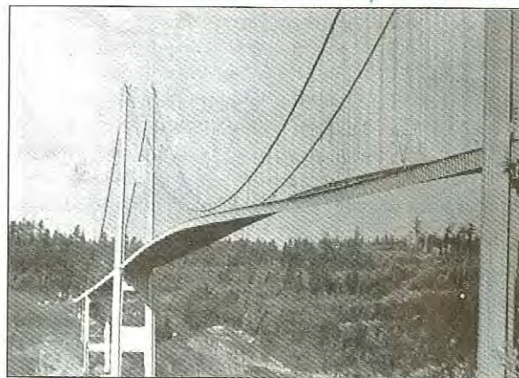
Figure 3: Aerolastic Instability of the Tacoma Narrow Bridge
